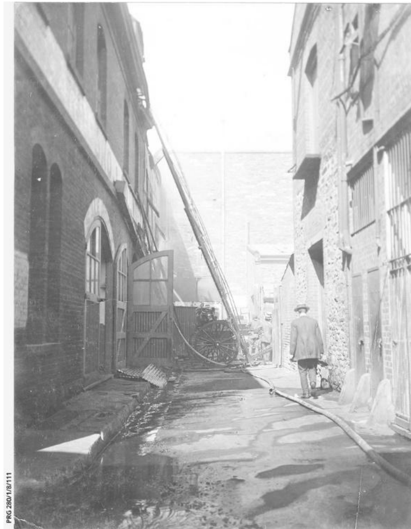
The aftermath of a fire at the premises of A.W. Sandford and Co. Ltd [PRG 280/1/8/111]. The aftermath of a fire at the premises of A.W. Sandford and Co. Ltd., produce salesmen and auctioneers, dairy machinery and refrigerating engineers, Imperial Place, Adelaide. 14 February 1914. Part of Searcy Collection
