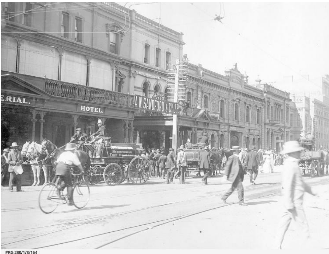
The State Library of South Australia, A fire at the premises of A.W. Sandford & Co. Ltd Produce Mart, Grenfell Street [PRG 280/1/8/164]. Horse drawn Metropolitan Fire Brigade vehicles, fire officers, and passers-by outside the premises of A.W. Sandford & Co. Ltd Produce Mart on Grenfell Street following a fire. 14 February 1914. Part of Searcy Collection
